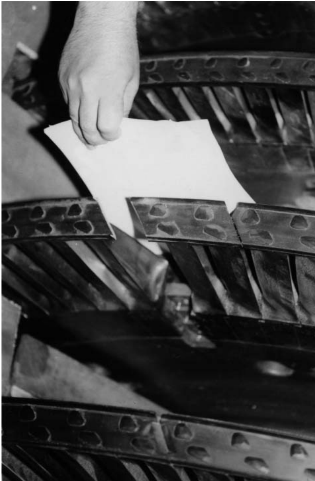
Fig. 3 The III-stage HP turbine shroud after the cutting and removal of the cracked blade
