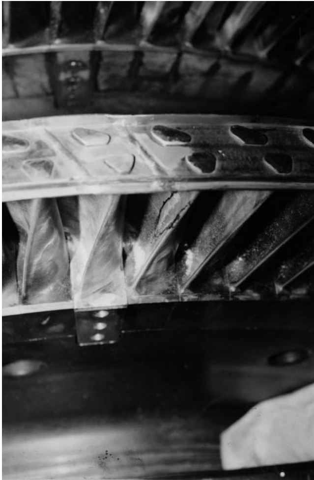
Fig. 5 The III-stage HP turbine shroud after in situ repair welding
